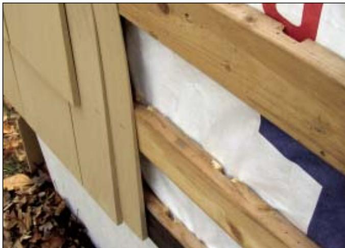
**FIGURE 1.** The author's first experiences with venting shingles relied on back-kerfed 1x3 furring strips. These back kerfs are essential for allowing water to drain out and air to flow between the horizontal strips, but cutting the kerfs with a dado blade in a radial arm saw proved too labor intensive.
