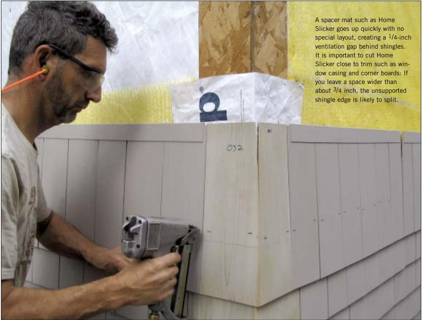
A spacer mat such as Home Slicker goes up quickly with no special layout, creating a 1/4-inch ventilation gap behind shingles. It is important to cut Home Slicker close to trim such as window casing and corner boards: If you leave a space wider than about 3/4 inch, the unsupported shingle edge is likely to split.
