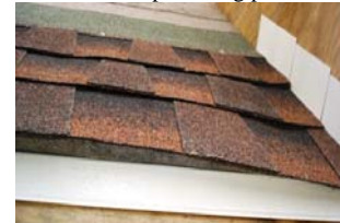
Step 7 ^ Continue by installing a starter course & shingles with a 1/2" to 1" overhang at the eaves edge. SmartVent End Caps are Patent Pending in the USPTO.
