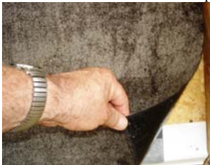
Step 5 ^ Install ice shield tight to the wall.
