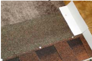
Step 7 ^ Continue by installing a starter course & shingles with a 1/2" to 1" overhang at the eaves edge. SmartVent End Caps are Patent Pending in the USPTO.
