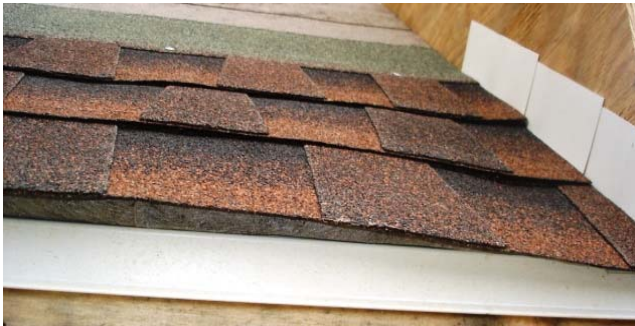
SmartVent End Cap after Installation (above). ^ Follow the steps below to achieve the required results. Ice shield installs on top of SmartVent & End Caps.
