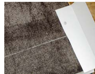
Step 6 ^ Install wall step flashing per code.
