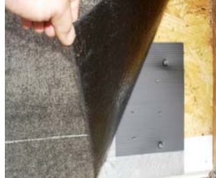
Step 4 ^ Install ice shield over SmartVent.
