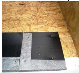
Step 2 (above) ^ and Nail end caps at four corners.
