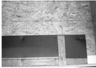
**Step 4-** Install 36" wide ice & water membrane only over the SmartVent™ and Universal Tapered End Cap tight against side wall and continuously across the roof. Keep 36" ice & water membrane flush to the SmartVent™ lift edge which will cover the entire top surface of the vent.
