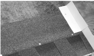
**Step 8-** Continue installing underlayment and shingles up the roof with step flashing. The Universal Tapered End Cap slopes the shingles down to the level of the wall flashing as shown.
