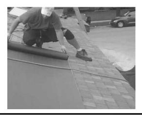
**STEP 7:** Install a starter course of shingle overhanging the SmartVent edge by at least 1/2" and not more than 3/4".
