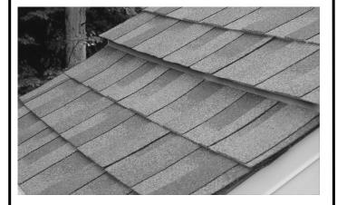
**STEP 8:** Install the shingles over the starter course and continue to shingle the roof normally.
