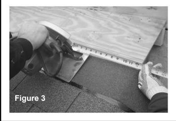
**STEP 4:** Remove the plywood decking after the continuous cut and ensure the airflow is unobstructed from the cut slit to the ridge or off-ridge exhaust vent.
