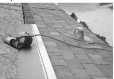
**STEP 6:** Apply a roll of ice and water membrane on top of the SmartVent and directly to the plywood above the SmartVent.
